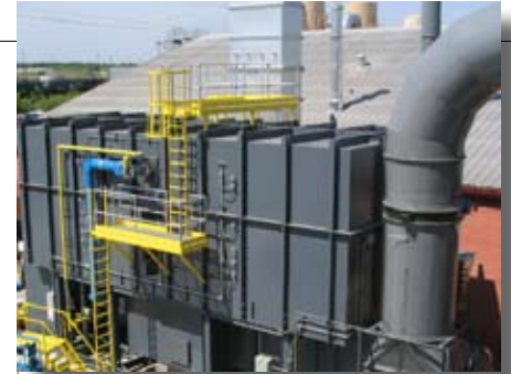
CLEANSWITCH® RTO unit for VOC treatment from flexible packaging plant
