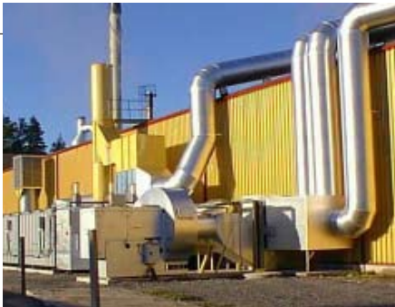
A VOCSIDIZER® RTO for VOC emissions from flexo printing processes and odours removal
